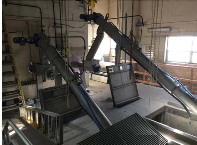
Work is scheduled to begin the week of January 29 on the grit system. The by-pass pumps and piping are being removed and excavation is scheduled to begin.
